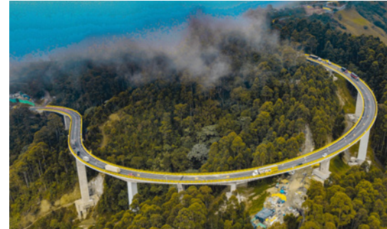
The horseshoe-shaped Yarumo Blanco Viaduct in Colombia significantly reduces travel time from Bogota to the Pacific. In front on the right at the bottom of the short pier, you can see the concrete cube under which the retrofitted isolators are located.
