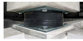
One of the 243 lead rubber bearings between the upper concrete platform and the lower concrete trough. Clearly visible are the ring-shaped deformations of the elastomer-steel plate layering.
