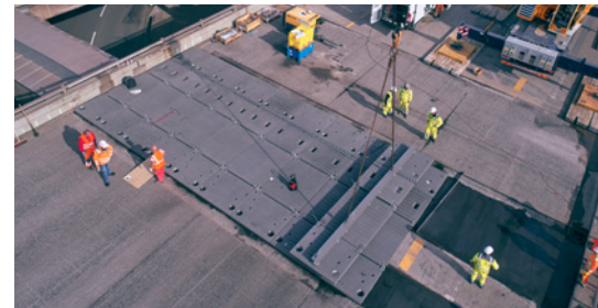
Lifting into position of a Mega-MMBS with a 100-t crane.
