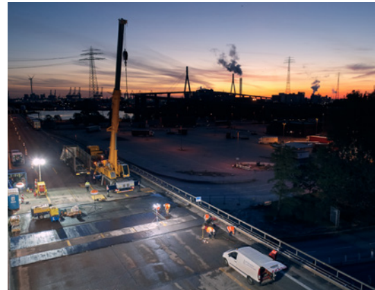
The work was done in three-shift operation 55 hours around the clock.
