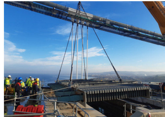
The MSM® Swivel Joist Expansion Joint during installation in the bridge.
