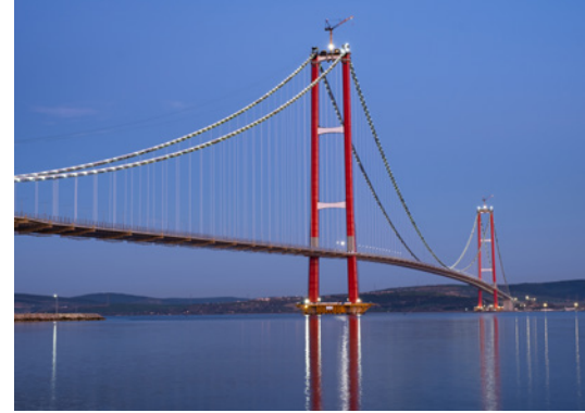
The world's longest suspension bridge, 1915Çanakkale over the Çanakkale Strait, has a main span of 2,023 metres.
