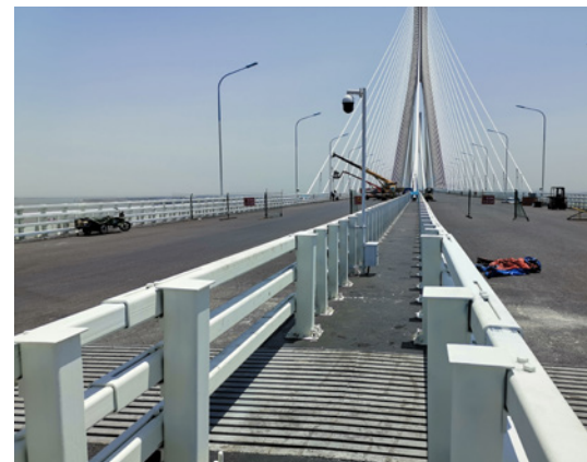
Upper deck of the double-decker Hutong Bridge north of Shanghai. The expansion joint was delivered in two parts and welded on site.
