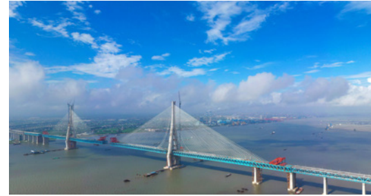
Record bridge in China: the Hutong bridge featuring a length of 11 km with the central cable-stayed bridge with a length of 1,092 m.
