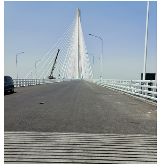
18 lamellae accommodate the expansion movements of the main bridge.
