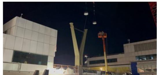
Installation of the SIP®-Bearings on top of the Y-columns. Work performed at night as the airport is being renovated while continuing to operate.
