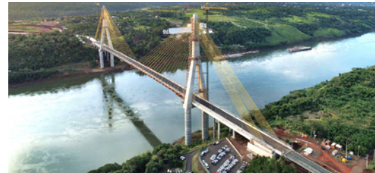
The friendship bridge between Brazil and Paraguay is due to be inaugurated in 2024.
