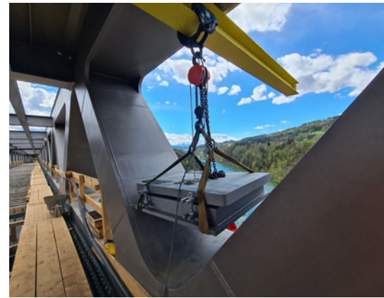
Lifting in the SIP® bearings using specific mounting girders.
