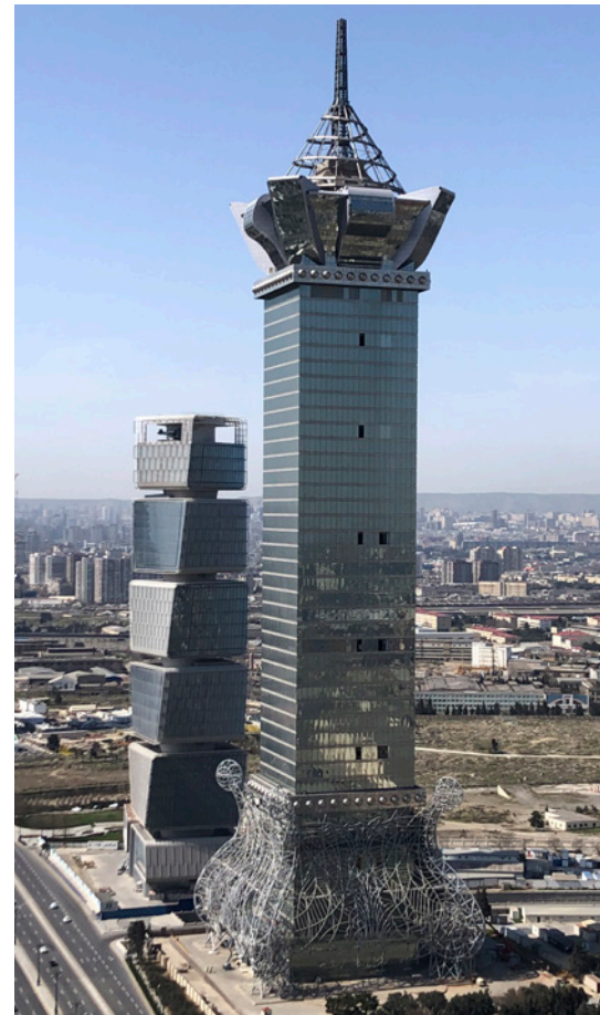
View on the Baku Tower: the vibration damper operates above the widest point of the crown.
