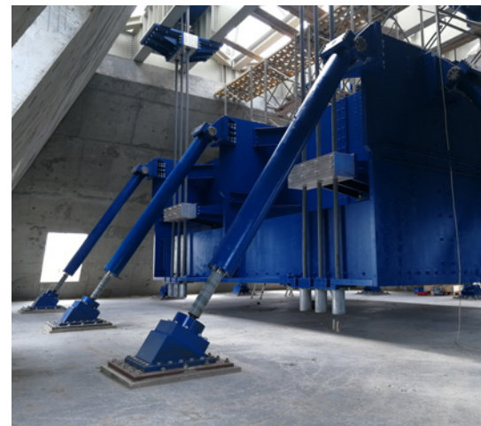
The complete TMD (Tuned Mass Damper) with diagonally docked hydraulic dampers that limit the amplitude to 1.3 m in case of an earthquake. Three pendulum cables at each of the four suspension points are manufactured as fully locked cables with a smooth surface.
