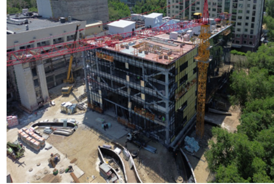
The SHARKS® can be seen on the front side of the extension building, shown here during construction. The right-hand facade has already been cladded. The main building, which is being renovated, can be seen on the left.
