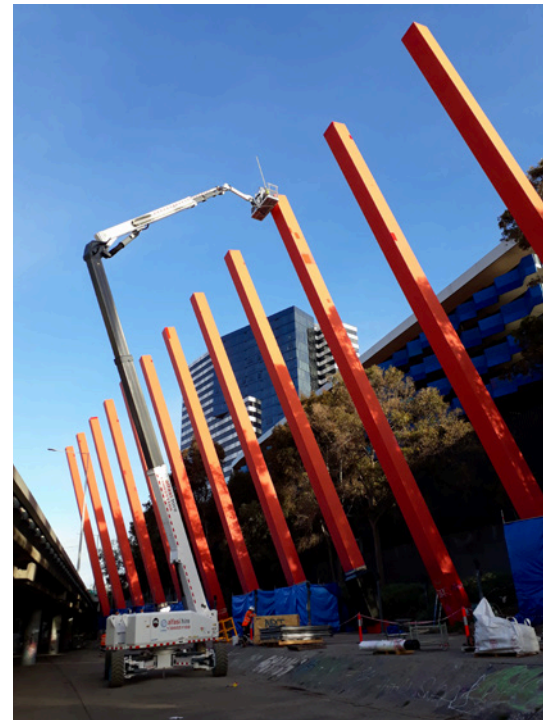
Installation of a new damper.
