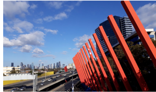
Red Sticks in Melbourne fitted with MAURER TMDs to minimise wind-induced structural vibrations.
