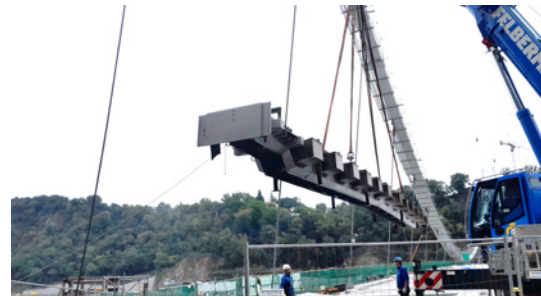
The expansion joint is hoisted into place in July 2023.
