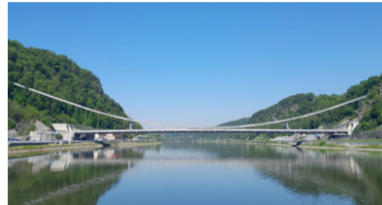
A true suspension bridge: the 500-metre-long suspension cables of the Danube bridge in Linz are anchored in the rock.
