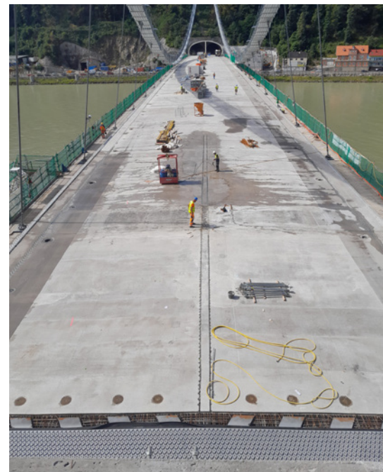
View from the crown of the tunnel along the entire Danube bridge. One of the expansion joints is visible at the bottom of the image.
