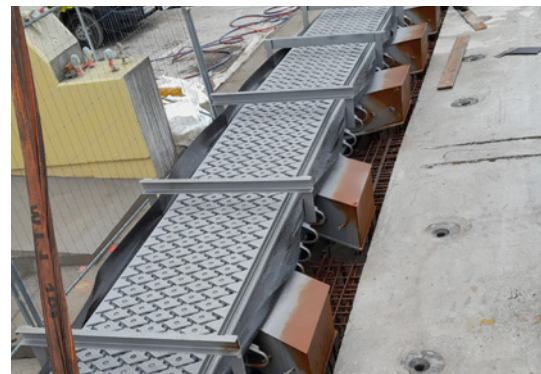
The expansion joint being fitted at the tunnel entrance. The image clearly shows the rhomboid plates welded on for noise reduction.
