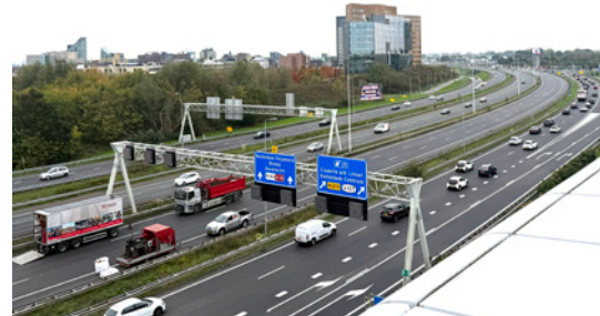
The 12-lane bridge with the s'-Gravenweg viaduct. The second bridge structure is closed, with the construction site vehicles visible on the left.
