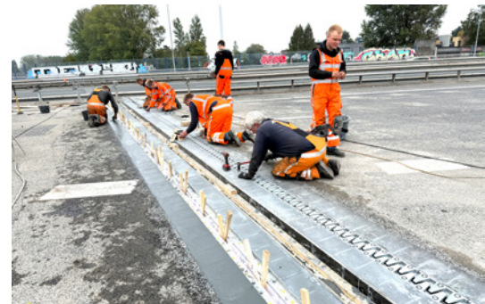
Two expansion joint constructions installed behind one another. The special steel fibre-reinforced concrete is being added to the one on the left, while the one on the right is being fitted with the noise reduction system.
