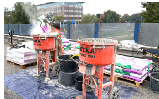
The special steel fibre-reinforced concrete is mixed on site.
