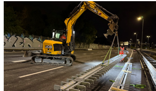
The expansion joints are placed down in the night ready for installation.
