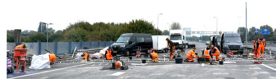
Meeting the tight schedule requires lots of installation workers.
