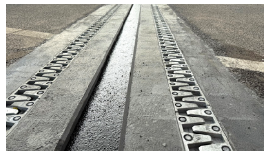
Two installed expansion joint constructions with noise reduction system. The gap in the middle will be filled by the last layer of asphalt.
