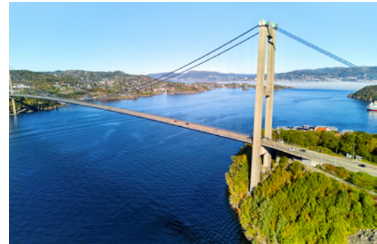
The Askøy bridge in south-west Norway has a main span of 850 m.
