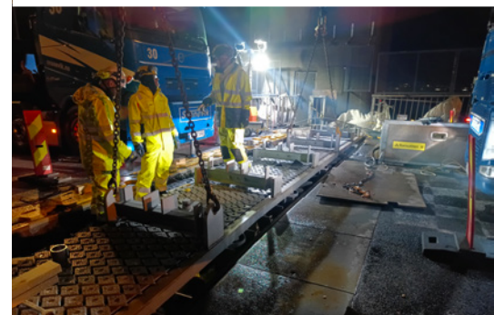
The new centre beam box is hoisted into place overnight.
