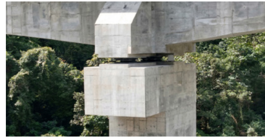
Bearings installed on one of the piers.
