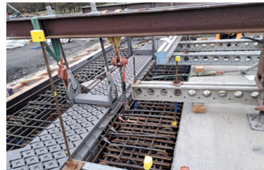
The expansion joint is installed before the pouring of concrete.
