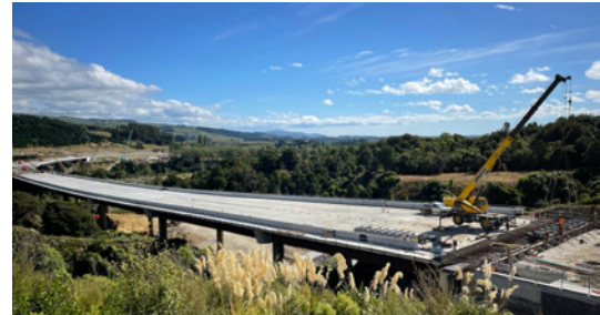
The EcoViaduct, with the open end without expansion joint visible on the right.
