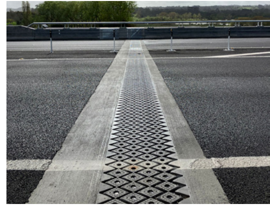
The fully installed expansion joint.
