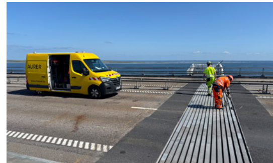
The finishing touches to the new expansion joint construction.
