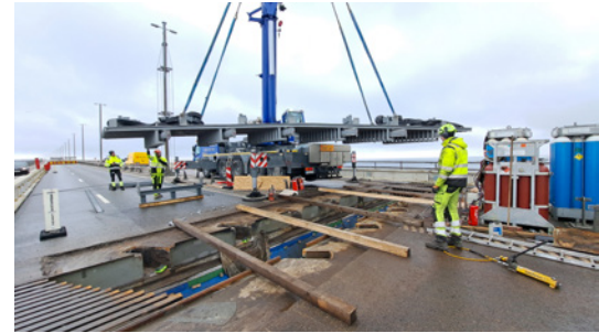
The central part of the first new expansion joint construction is lifted into place. Traffic continues to pass by to the right and left.
