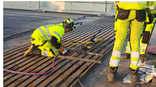
Preparations for removing the old expansion joint construction.
