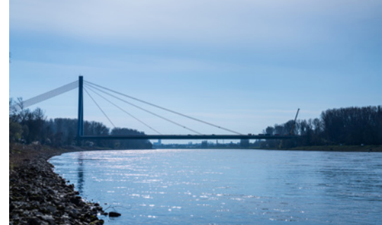
The A61 bridge over the Rhine at Speyer. The expansion joint between the asymmetrical cable-stayed bridge and the approach bridge on the right was replaced.
