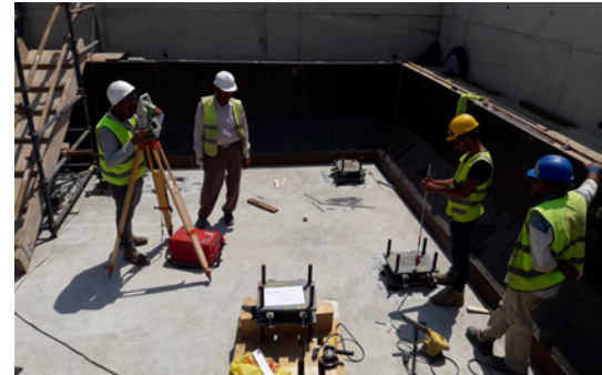
Installation of the lead rubber bearings.
