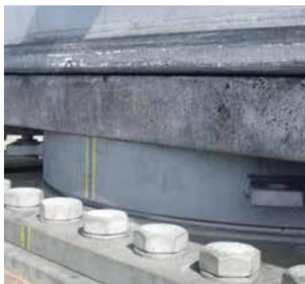
The bearings underneath the Bogibeel Bridge transmit a load of 2,800 t in the smallest of spaces.
