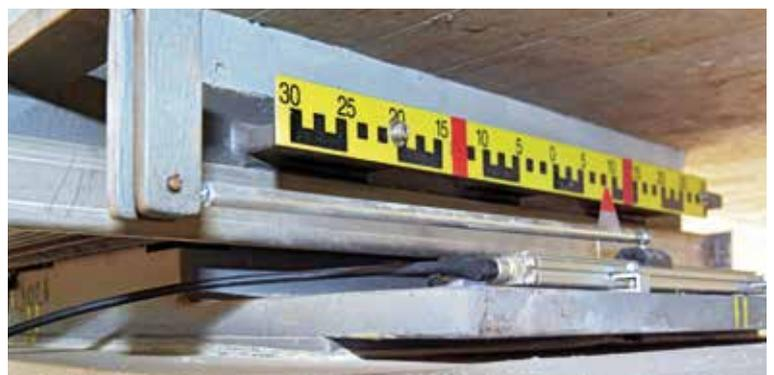
Spherical sliding bearing KGA with displacement measuring
