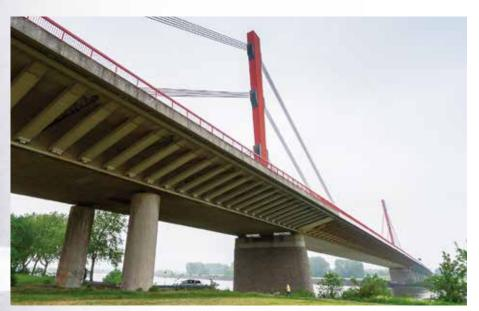
The two steel pylons of the cable-stayed bridge have a height of 66.7 m and are located in the center axis of the bridge. On each side, three harp-shaped cable groups are anchored in the pylons.
