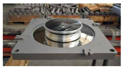
Lower sliding surface with articulated slider
