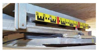
Spherical sliding bearing KGA with displacement measuring
