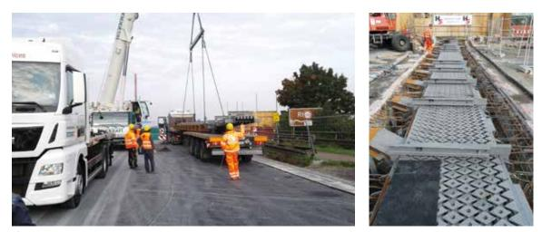
The new expansion joints are noise-reduced. When crossing the roadway expansion joints, you will not recognize any difference to the road surface.
