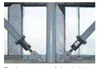
The dampers are installed at the bottom end of the cross braces. They have a length of 750 mm.
