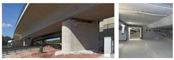
Instrumented bearing at axis 40. On the right: view into the box girder of the bridge, in the foreground sensor cables
