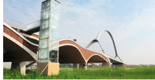
The new Stadsbrug in Nijmegen: Arch bridges in the approach and a combined steel arch suspension bridge for the main spacing.
