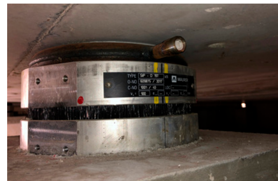
One of the Typ SIP®-D-type double sliding isolation pendulums: They have an upper and lower curved sliding surface.
