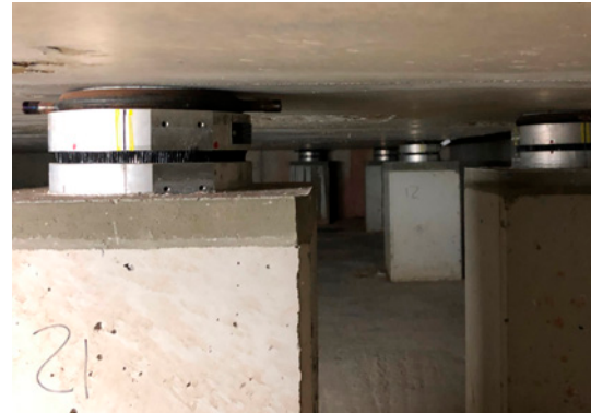
The historic farmhouse stands on 45 supports on which the isolators rest.
