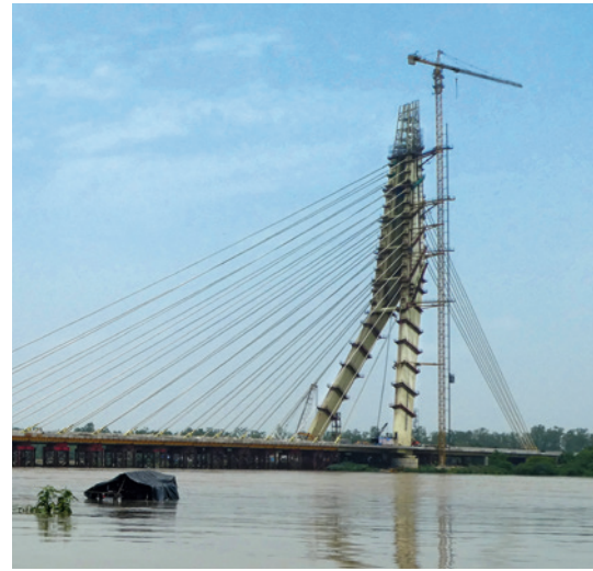
The Signature Bridge in Delhi in summer 2018.
