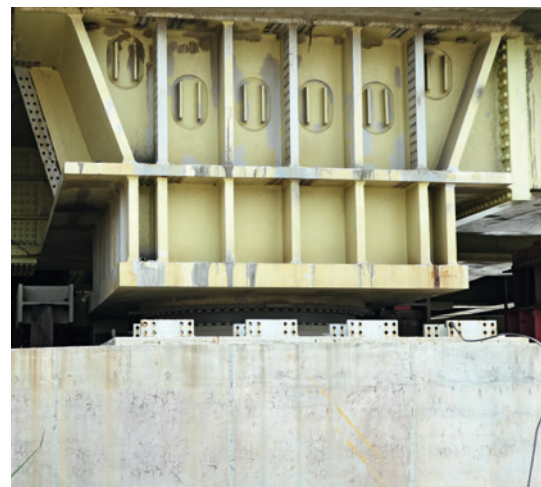
The largest CE-marked MSM® spherical bearing ever built with a structural load of up to 231,000 kN under one of the two pylon footings.
