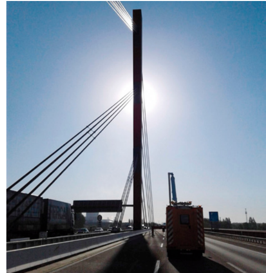
Two 66.7 m high steel pylons bear the main load of the Baerl Rhine Bridge. Traffic guidance 4 + 0: four traffic lanes on the left, completely closed on the right.
