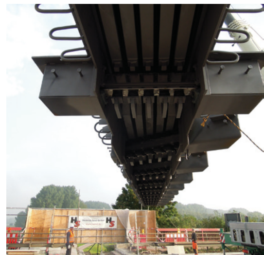
Lifting an expansion joint into position with a 100-t crane.
