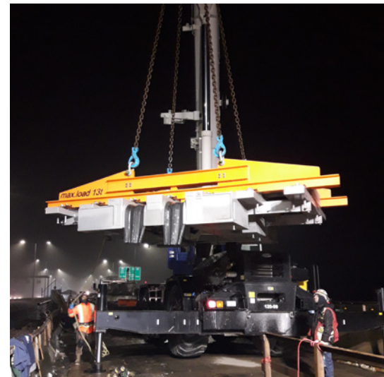
Installation of the first Guided Cross-Tie in Montreal in November 2020.
