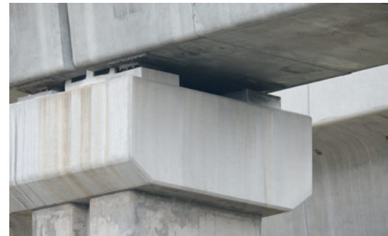
Each single-span beam rests on four bearings.
