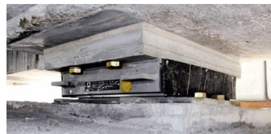
The picture shows a longitudinally sliding guide bearing designed for a structural load of up to 6 MN.
