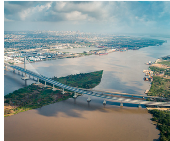
Pumarejo cable-stayed bridge near Barranquilla, the longest road bridge in Colombia.
