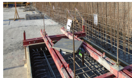
Bearing plate during installation in 2019.
