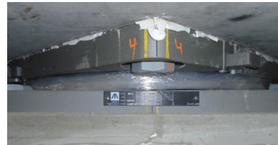
Installed bearing in 2021.
