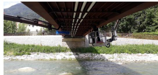
From two sides, the crane jibs service the place of assembly at the bridge center: the damper is shown on the left, the fitters in the basket on the right.
