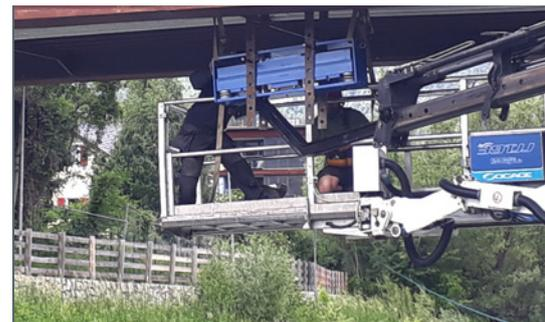
Four perforated metal plates are vertically welded on as an auxiliary device for proper positioning of the damper. The crane pushes the damper upwards, hole by hole, alternating on the right and on the left; the plug-in rods secure the respective position.
