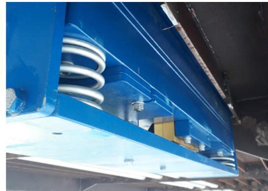
Once the dampers are firmly bolted, the perforated metal plates are removed.
