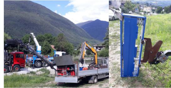
Left: Each of the two crane trucks in the background was used to hoist one assembly basket and one damper underneath the bridge.
