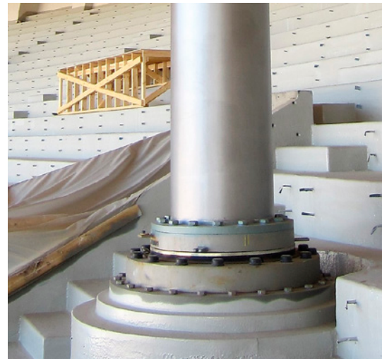
One of eleven uplift spherical bearings: at a bearing diameter of up to 1,500 mm it accommodates alternating loads from -12.000 kN pressure up to +3.000 kN tension and allows virtually restraint-free rotation under horizontal loads.
