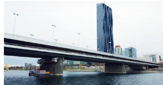
Pier P7 of the Reichsbrücke in Vienna during the replacement works. In the background the 220m high Danube City Tower with the unique semi-active dampers, that respond to various load cases, made by MAURER too.
