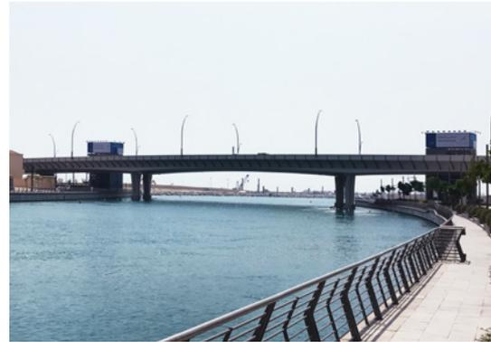
At first glance this is a bridge like any other. But it is one of the drei bridges over the Dubai Water Canal for which as a worldwide first time a sliding material was specified that had to be proven for 60°C and 40 MPa.
