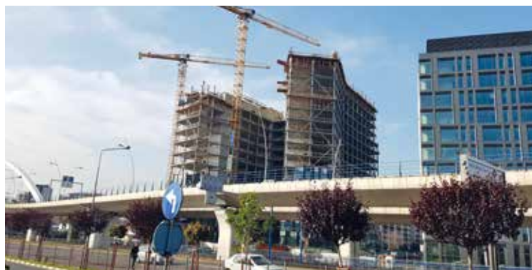
Fig. 6: Installed devices within Basarab Overpass in Bucharest
