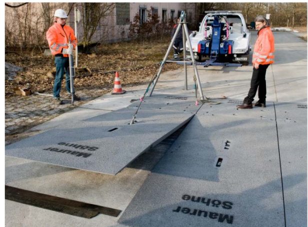
Fig. 2 - Opening with wrench and tripod
