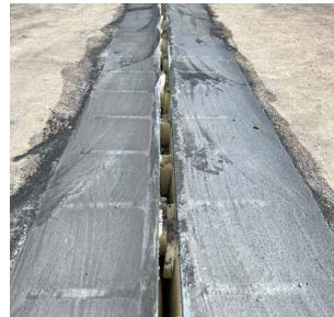
Anchorage with steel fiber concrete
