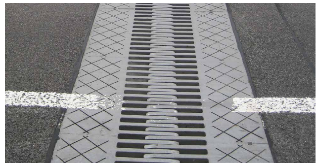
Welded finger joint (FW)
