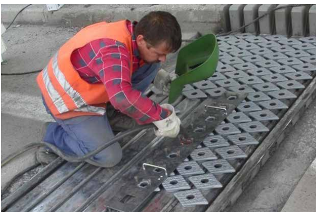
Tacking of the rhombic elements
