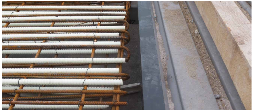
Clamped edge profile protection
