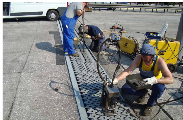
Welding of the rhombic elements with robot
