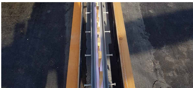
Compact Expansion Joint with Betoflex®-anchorage as longitudinal joint between two superstructures
