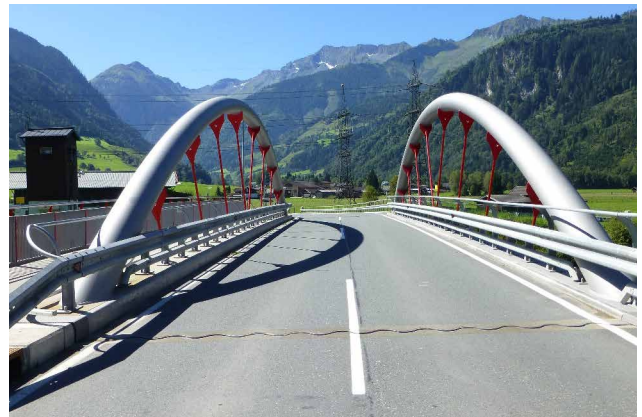
L264, Salzach Bridge Uttendorf, Austria: Expansion joints D1-B and XW1 with Betoflex® header
