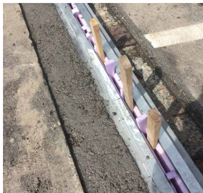
Header grouted on one side
