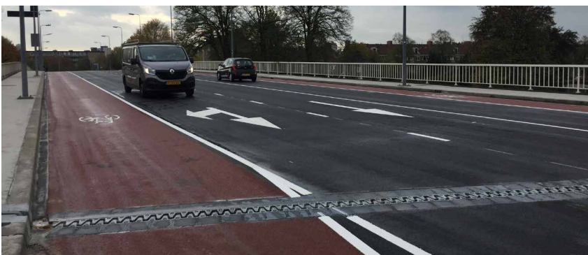
XC1-B joint installation examples
