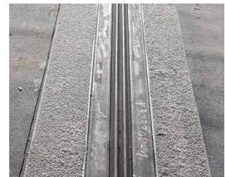
Compact expansion joint with Betoflex®
