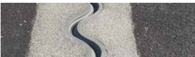
Noise-reduced XW1 expansion joint with polymer concrete Betoflex®
