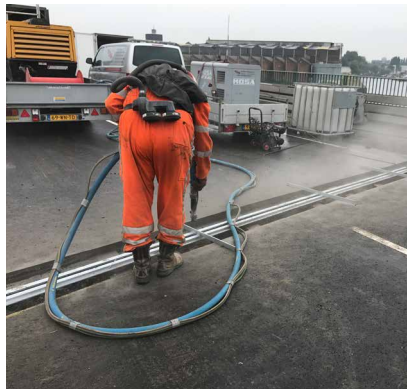
Abrasive blasting of the connection surfaces
