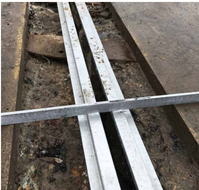
Aligning of the expansion joint
