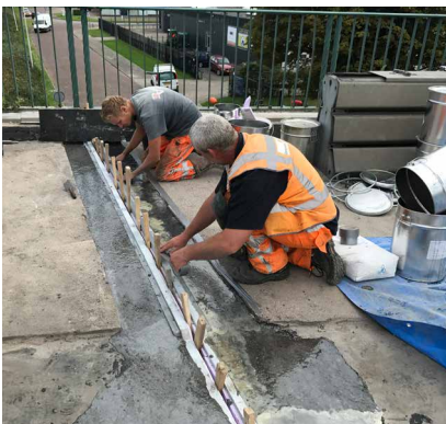
Fixing the gap width
