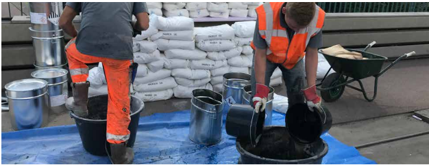
Mixing of Betoflex® on site
