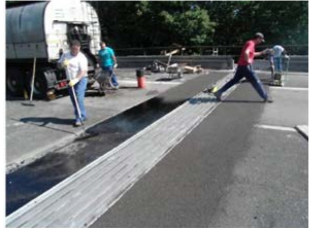
Fig. 9 - Placement of mastic asphalt
