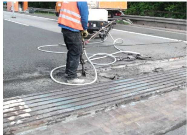
Fig. 5 - Removal of cover layer, protection layer, and waterproofing
