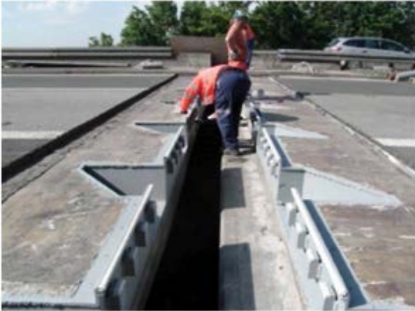
Fig. 7 - New corrosion protection of the remaining part of the expansion joint
