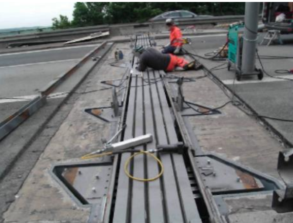
Fig. 8 - Welding of the new expansion joint into the old structure
